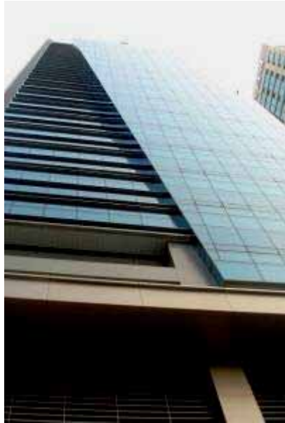
The 24-story Luther Tower
