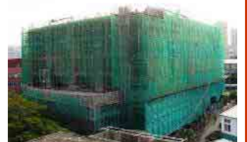
China Lutheran Seminary's building project has reached the 8th floor.
