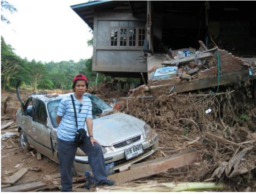
Photo 28: Northern flood damage
