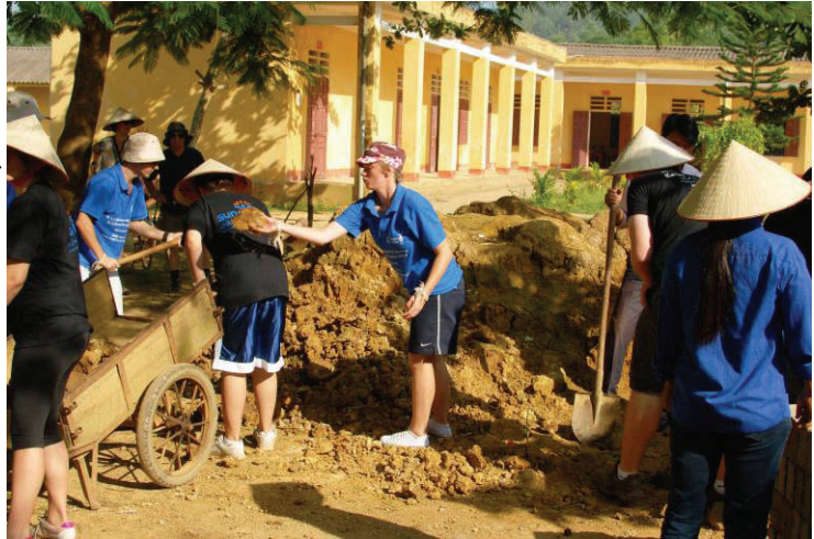
Kormilda students work hard to help level the ground at a primary school on a recent service trip
